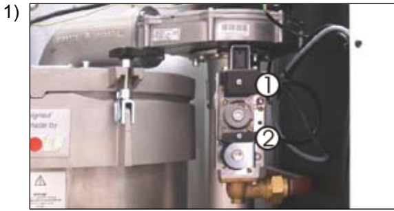
1) Unplug the connector ① ② (first undo Phillips head screws)
