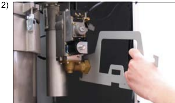
2) Undo gas connection at the gas combination valve
