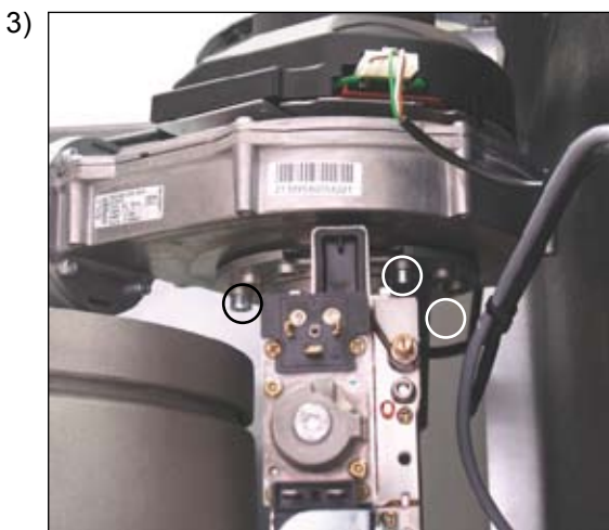
Undo the mixing chamber from the fan (three Allen screws 5 mm), and remove air inlet pipe where necessary.
