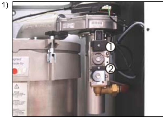
Unplug the connector ① ② (first undo Phillips head screws)
