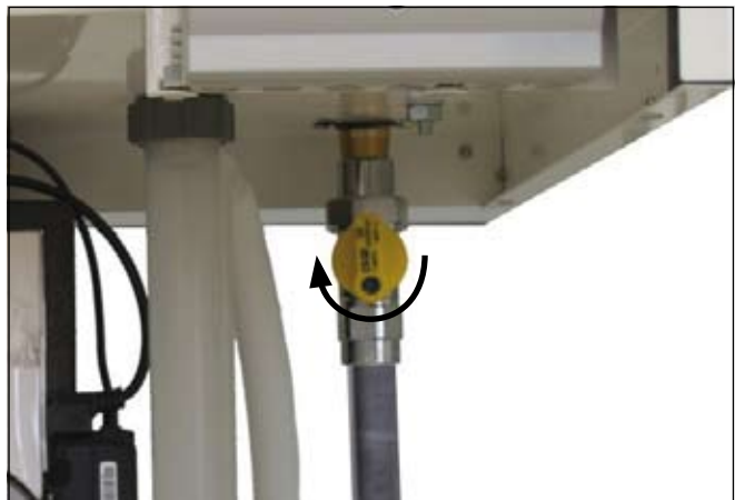
Figure: Gas connection
